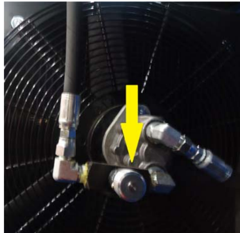
Figure 11: Oil cooler fan
