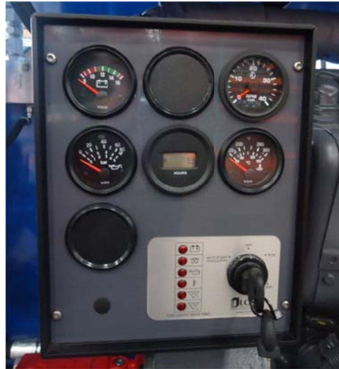
Figure 8: Electric LOFA start control panel
