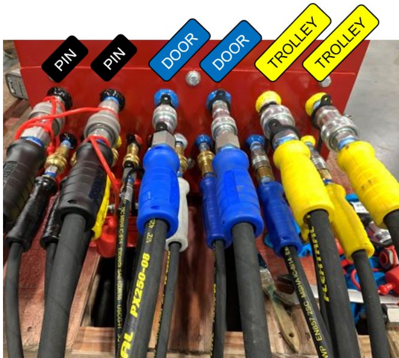
Control Console Supply & Return Connections
